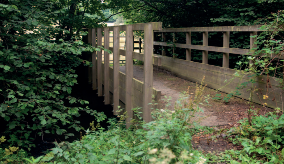
Bridge over Thornton Beck at mile 45.5
