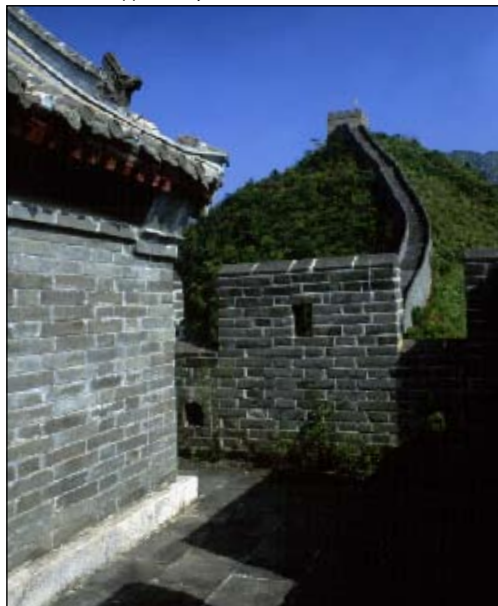
View from the upper storey of a watch-tower
