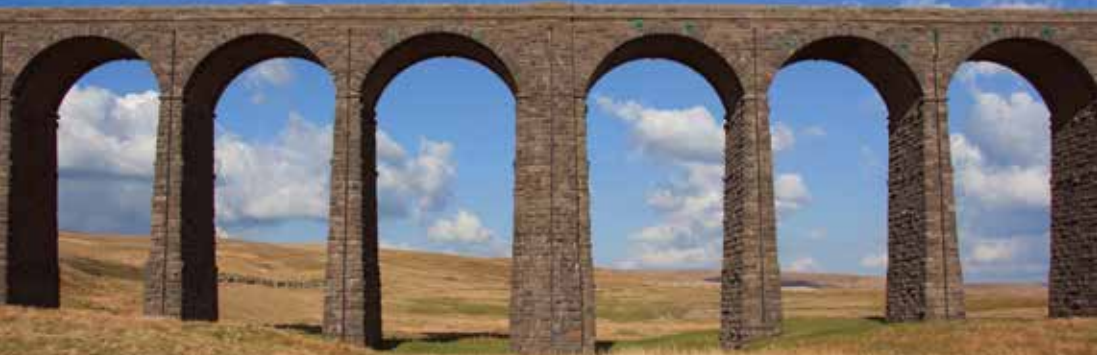
Ribblehead Viaduct: the central six arches
