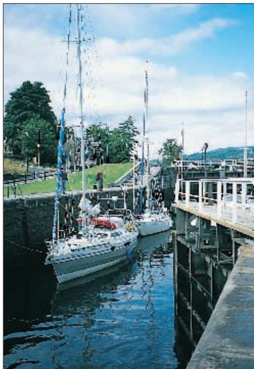
Lock gates opening at Fort Augustus
